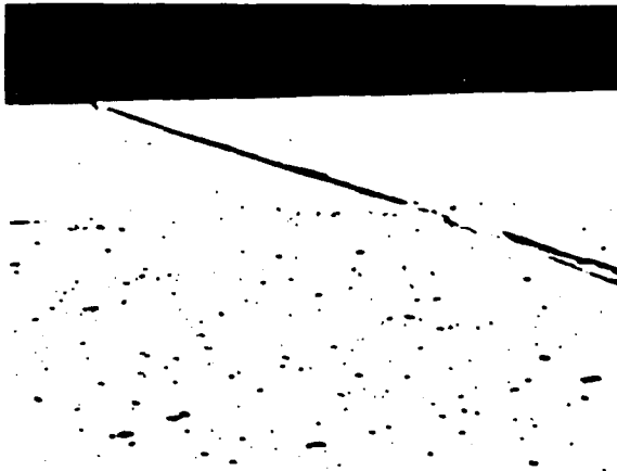
Fig. 3.2.1.2 — Aggregate pop-outs
